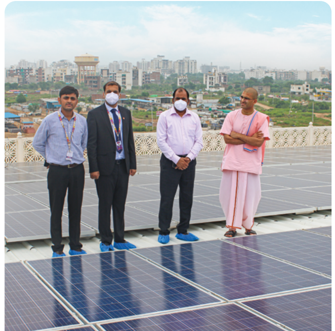
Supporting a greener planet with solar power grid installation
